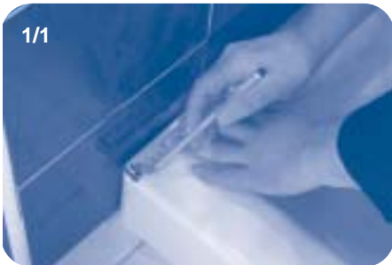
Fit wall brackets (A) 10mm in from the outside of the shower tray ensuring the profile is square. Mark each hole for position.
