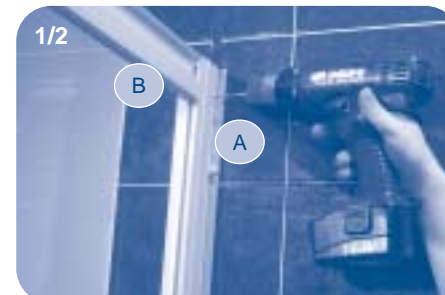
Ensure that the door is square within the frame and drill through existing holes in the door frame into fixed Wall Brackets (A) top and bottom.
