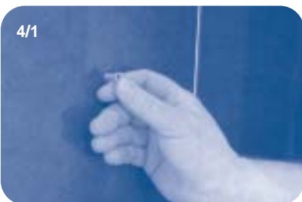
Insert wall plugs into drilled holes.
