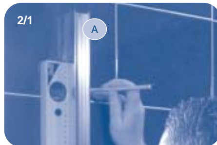
Fit wall brackets (A) 10mm in from the outside of the shower tray ensuring the profile is square. Mark each hole for position.
