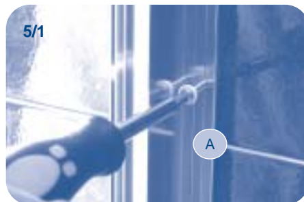
Insert 38mm screw into collar X 3 and secure one wall bracket to wall on the side the door will hinge from.
