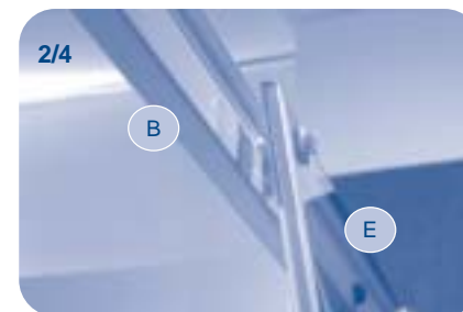
Hang Sliding Doors (E) onto Fixed Panels (B) by hooking wheels onto track.
