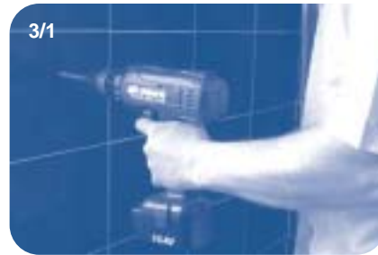
3/1 Drill with a 5.5mm masonry drill bit.
