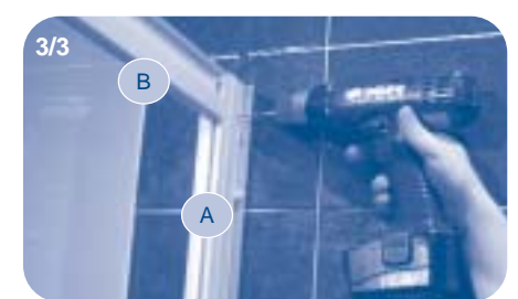
3/3 Ensure fixed panels are square, drill through existing hole in Fixed Panels (B) into fixed Wall Brackets (A) top and bottom.
