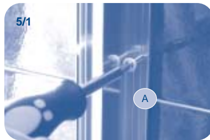
5/1 Insert 38mm screw into collar and secure both wall brackets to wall.
