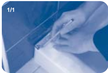
1/1 Fit wall brackets (A) 10mm in from the outside of the shower tray ensuring the profile is square. Mark each hole for position.
