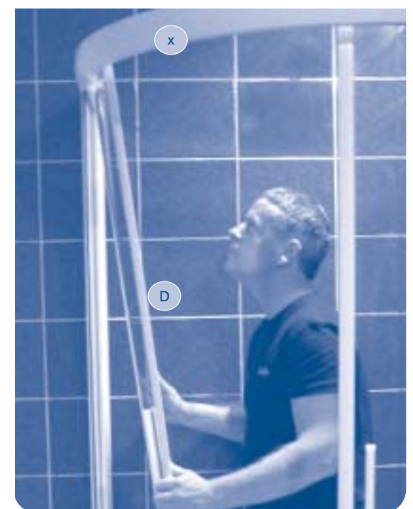
Secure Sliding Door (E) onto Fixed Panels (B) by turning the knob anti-clockwise until you hear a click. The screw can be loosened for ease of turning, retighten afterwards.
