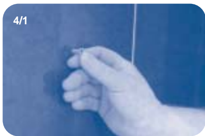
4/1 Insert wall plugs into drilled holes.
