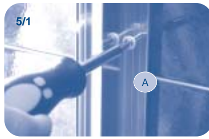
5/1 Insert a 38mm screw into collar x 3 and secure one wall bracket on the side where the fixed panel will be
