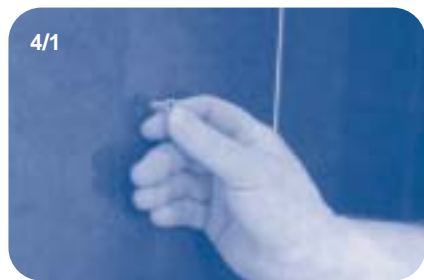
4/1 Insert wall plugs into drilled holes.
