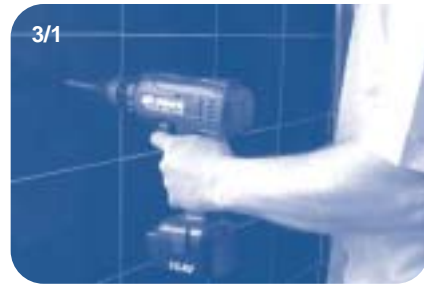
3/1 Drill with a 5.5mm masonry drill bit.
