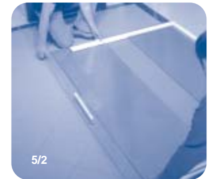
Slide door in to place as shown carefully aligning wheels on to track
