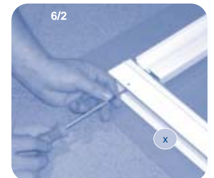
6/2 Secure Door Jamb with 4x35mm screws
